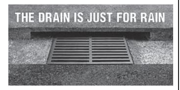
Storm water runoff from urban areas can carry pollutants and trash into the storm water drainage system. Water that flows down the drains in our homes first goes to sewage treatment facilities before it's released to bayous and rivers. But, water that flows into our storm water drainage system, along with other substances it collects, goes directly into our bayous, rivers, and ultimately into Galveston Bay. Unlike sewage, storm water receives no treatment.
