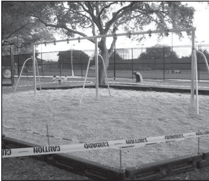
Check out the new Swing Set installation under construction in McDonald Park!
