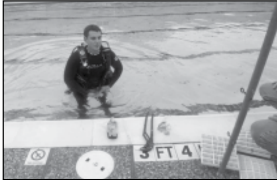
Picture above: scuba diver, Justin Martindale, fixing the pool's drain
