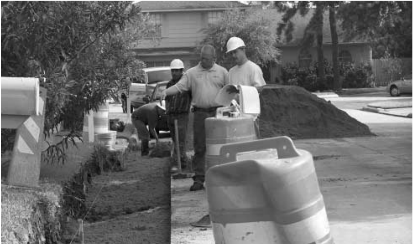
Public Works Director, Dan McGraw discusses street repairs that are in progress at several locations in the city
